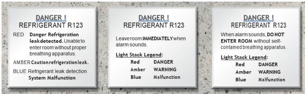
SIGN 1 to be installed beside the stackable flashing beacon inside the mechanical room
